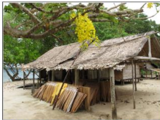
"A village house with a new Sago palm leaf roof ready to be installed, Nughu Island, Central Province" by Department of Foreign Affairs and Trade is licensed under CC BY 2.0.
